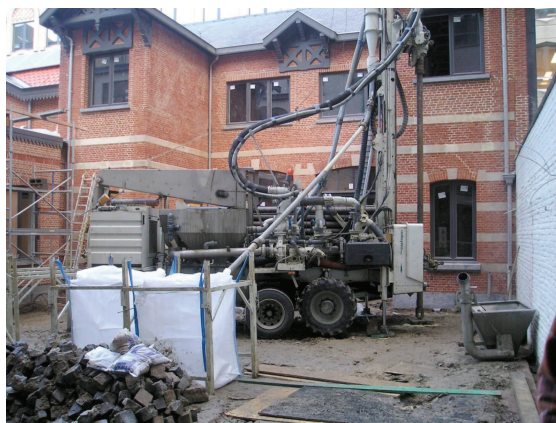
Fig. 6.27. Drilling rig inside the courtyard in Rue d'Arlon
