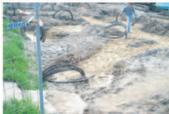
Fig. 6.25: Finished borehole heat exchangers, before connection
